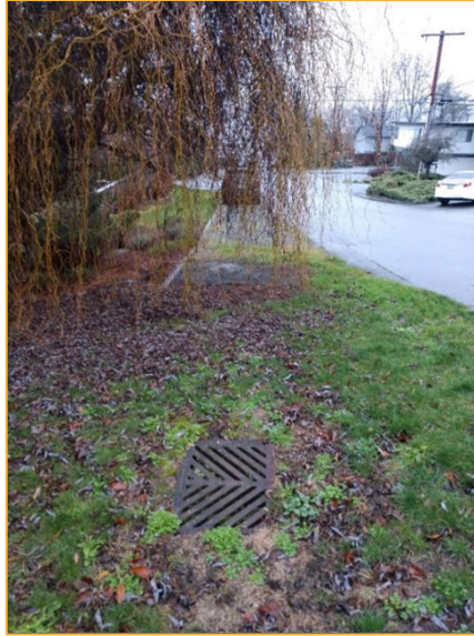
Photo N5 – Facing west along SE 28 th St approximately 95 feet west of Photo N4. Runoff is conveyed via this catch basin on the south side of the street toward Lake Washington.
