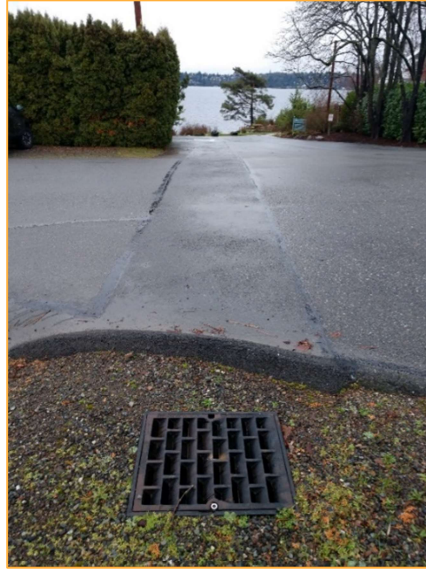
Photo N9 – Facing west along SE 28 th St approximately 95 feet west of Photo N8 at southeast corner of the intersection of SE 28 th St and 60 th Ave SE. Runoff is conveyed via this catch basin on the south side of the street toward Lake Washington.
