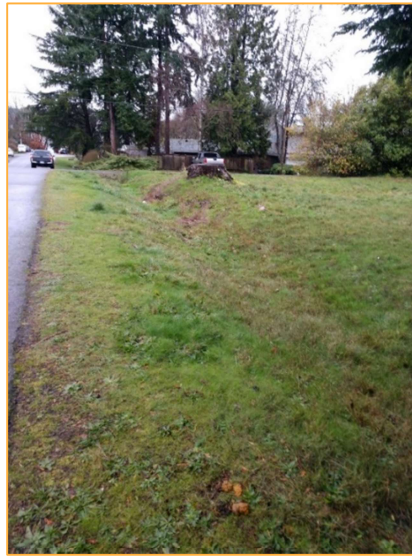
Photo S3 – Facing west along the north side of SE 30 th St approximately 35 feet west of Photo S2. Onsite runoff sheet flows in the southwestern direction to the ditch above and is conveyed west toward Lake Washington.
