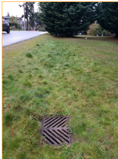
Photo S2 – Facing west along the north side of SE 30 th St approximately 55 feet west of Photo S1. Onsite runoff sheet flows in the southwestern direction to the catch basin above and is conveyed west toward Lake Washington.
