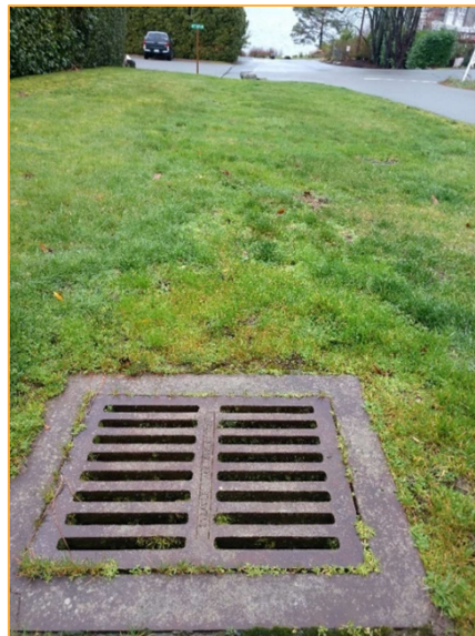
Photo N8 – Facing west along SE 28 th St approximately 40 feet west of Photo N7. Runoff is conveyed via this catch basin on the south side of the street toward Lake Washington.
