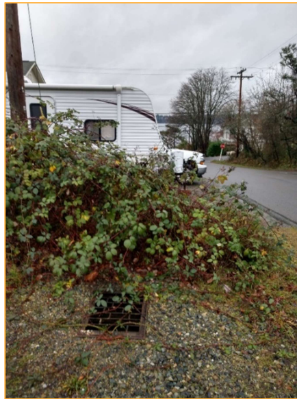
Photo N7 – Facing west along SE 28 th St approximately 90 feet west of Photo N6. Runoff is conveyed via this catch basin on the south side of the street toward Lake Washington.
