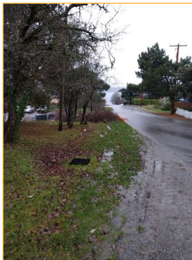
Photo N2 – Facing west along SE 28 th St approximately 170 feet west of Photo N1. Runoff continues to sheet flow northwest towards the conveyance system on the south side of the street.
