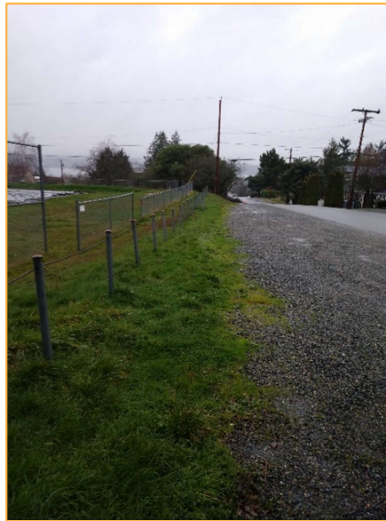
Photo N1 – Facing west along SE 28 th St. Onsite runoff sheet flows northwest toward the conveyance system on the south side of the street.
