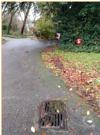
Photo S12 – Facing west in front of the entrance to Garfield Landing approximately 35 feet west of Photo S11. Runoff is conveyed west toward Lake Washington.
