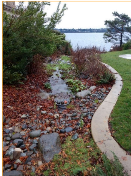
Photo N11 – Facing west in Calkins Landing. Runoff discharges via a pipe with a trash rack to a ditch upstream of the outfall to Lake Washington.
