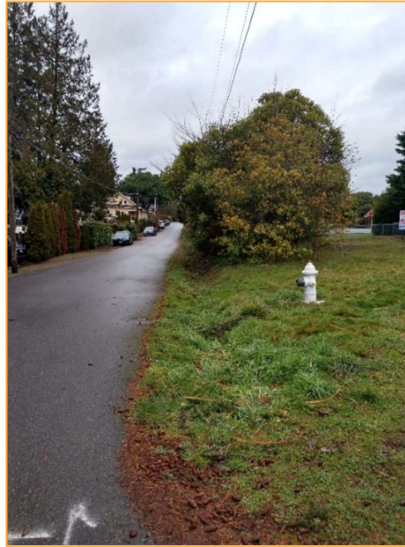
Photo S5 – Facing north on the east side of 62 nd Ave SE approximately 365 feet from Photo S4. Onsite runoff sheet flows in the southwest direction toward the ditch above and is conveyed south to be combined with the south basin downstream conveyance system.
